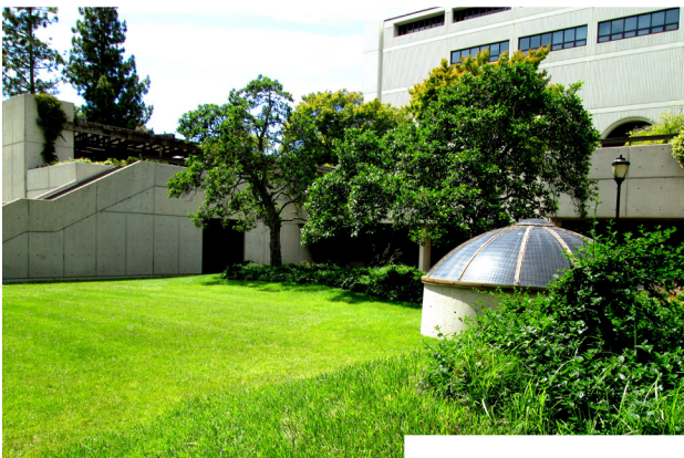
Left: Green roof at Bechtel Hall. Below Left: Native grasses on top of Li Ka Shing. Below: Aerial view of Li Ka Shing's extensive green roof, covered in a layer of vegetation.
